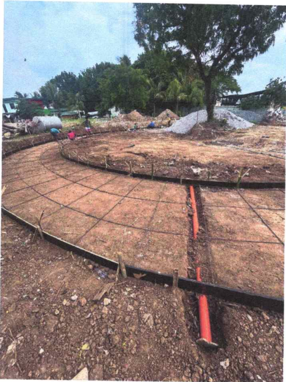
Construction of Pathway (Stampcrete)
